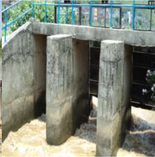
Irrigation canal in Butwal
