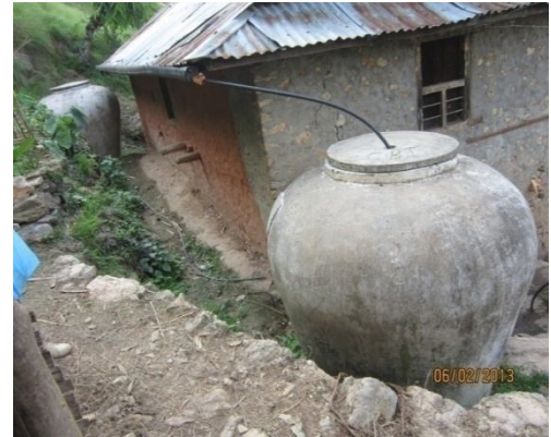
Picture 2: Cemented tank to collect Rain water
