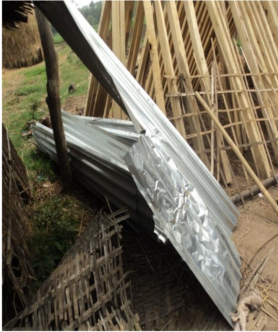
Photograph 9 : Cottage destruction by Elephants.
