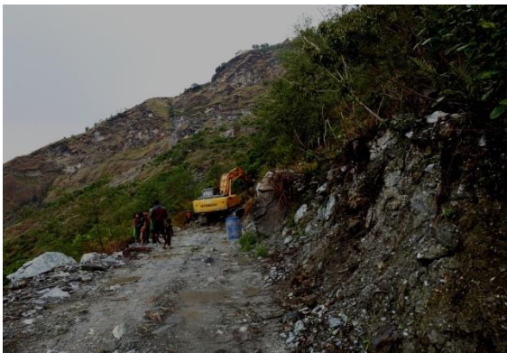
Photo 5: Road construction in Cheer's habitat
