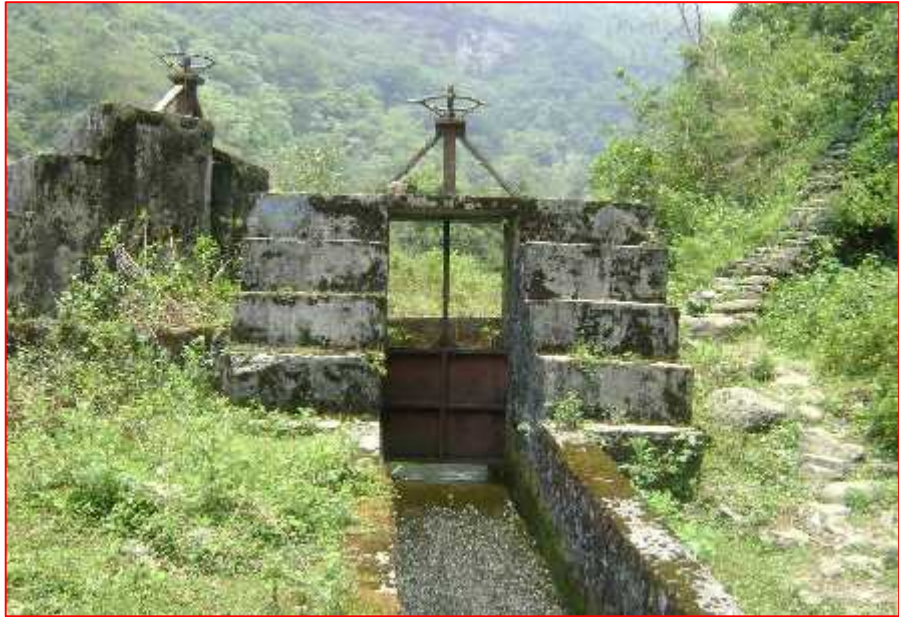
Photo 4.2: Glance of Shardikhola head works
