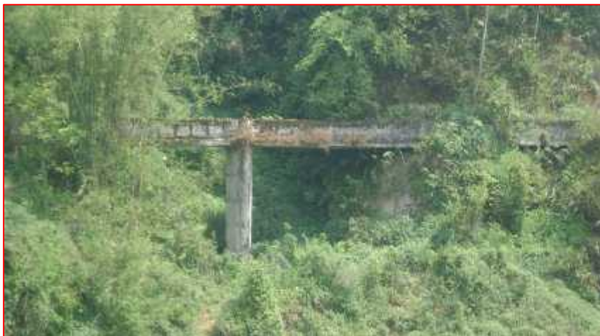
Photo 4.3: Culvert Bridge over Bhurjungkola
