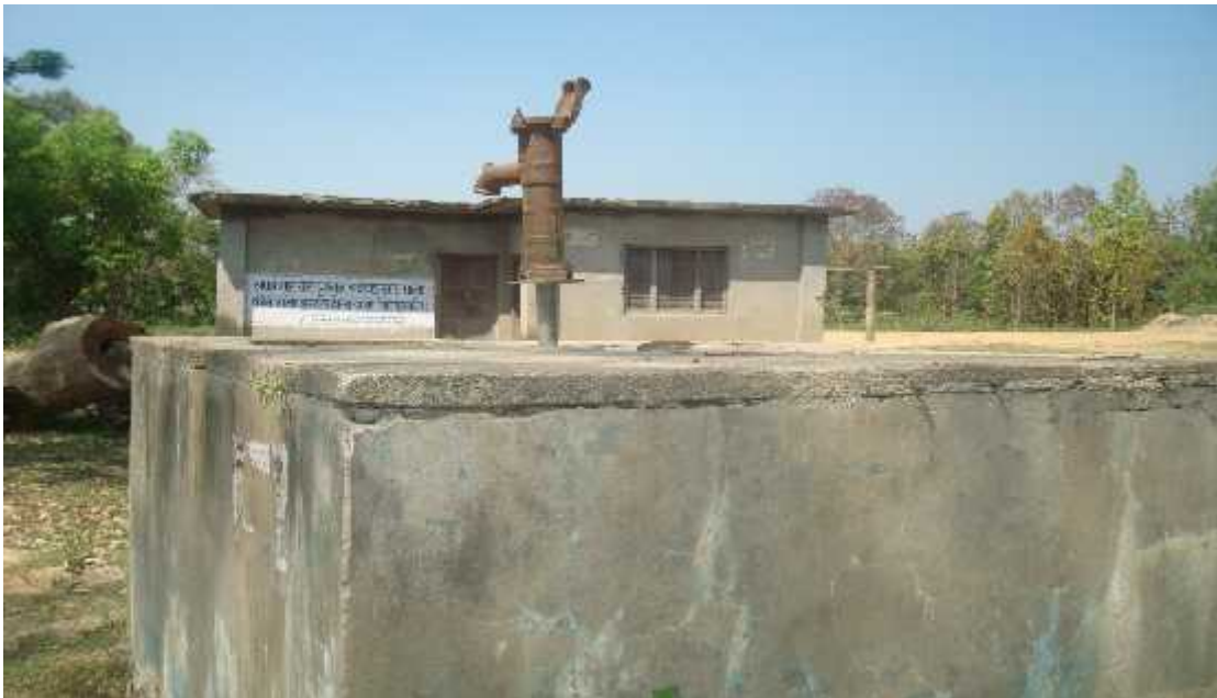
Photo- 2 CF office building with water storage tank for users
