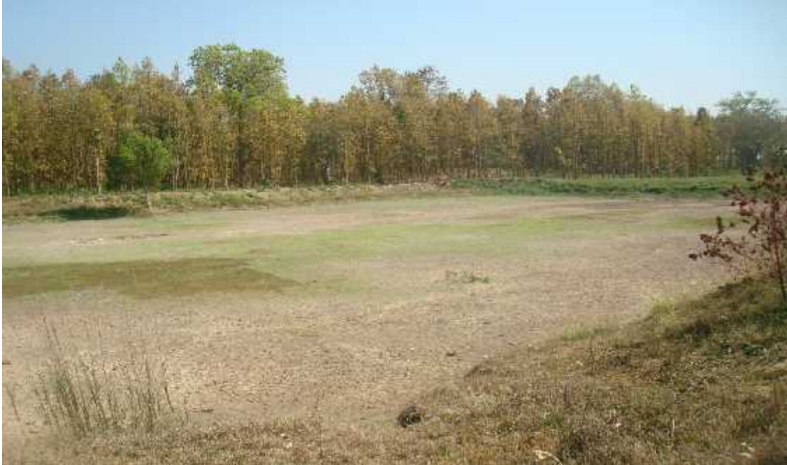
Photo- 5 Construction of recreation site (lake under construction)
