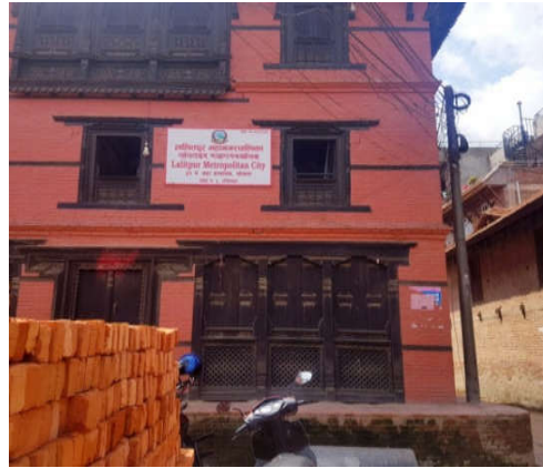
Picture 2: Ward office in Khokana village
