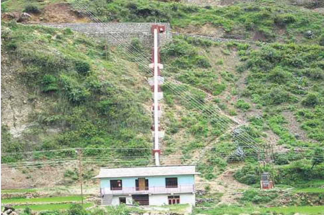
Nishi Khola II Micro Hydro Project Boharagaun -9, Baglung.
