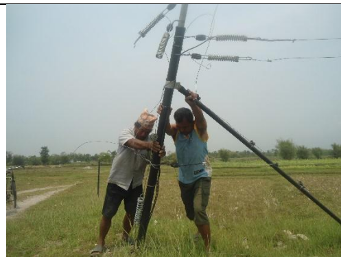
Photo 4. Technicians maintaining electric fence
