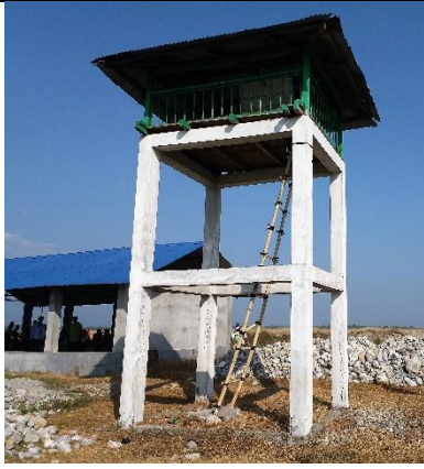
Photo 9. Newly constructed watch tower (toong)
