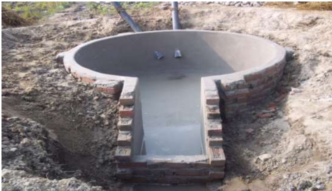
Photo 4 : Under construction biogas plant at study area
