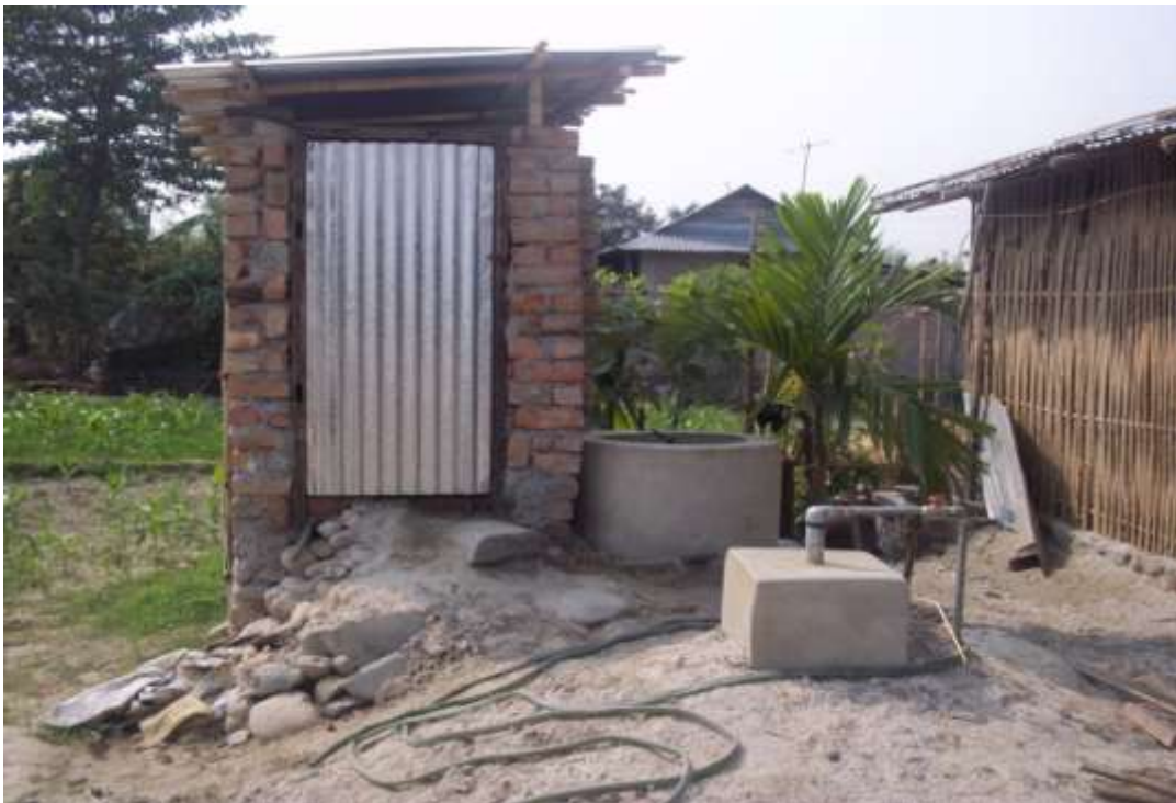
Photo 6 : Toilet attached biogas plant at study area
