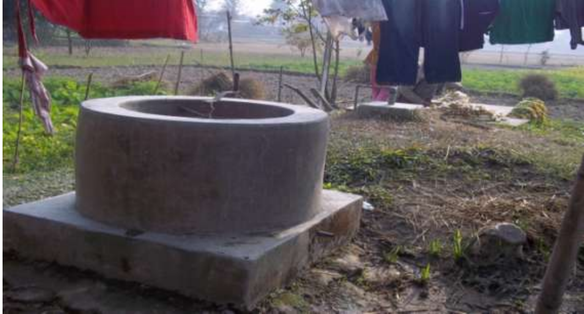
Photo 1: Newly constructed BGP at study area
