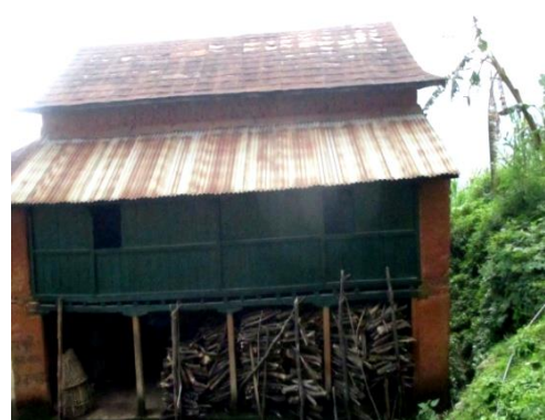
f. Piles of firewood inside the house
