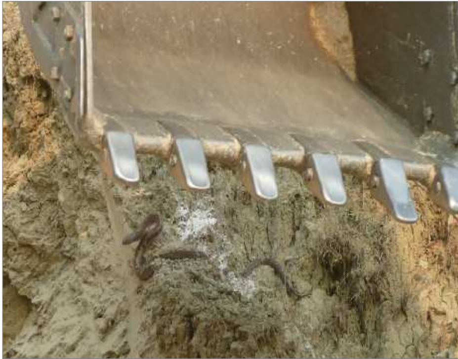
Fig 6.7. Cobra in trench killed by the excavator.
