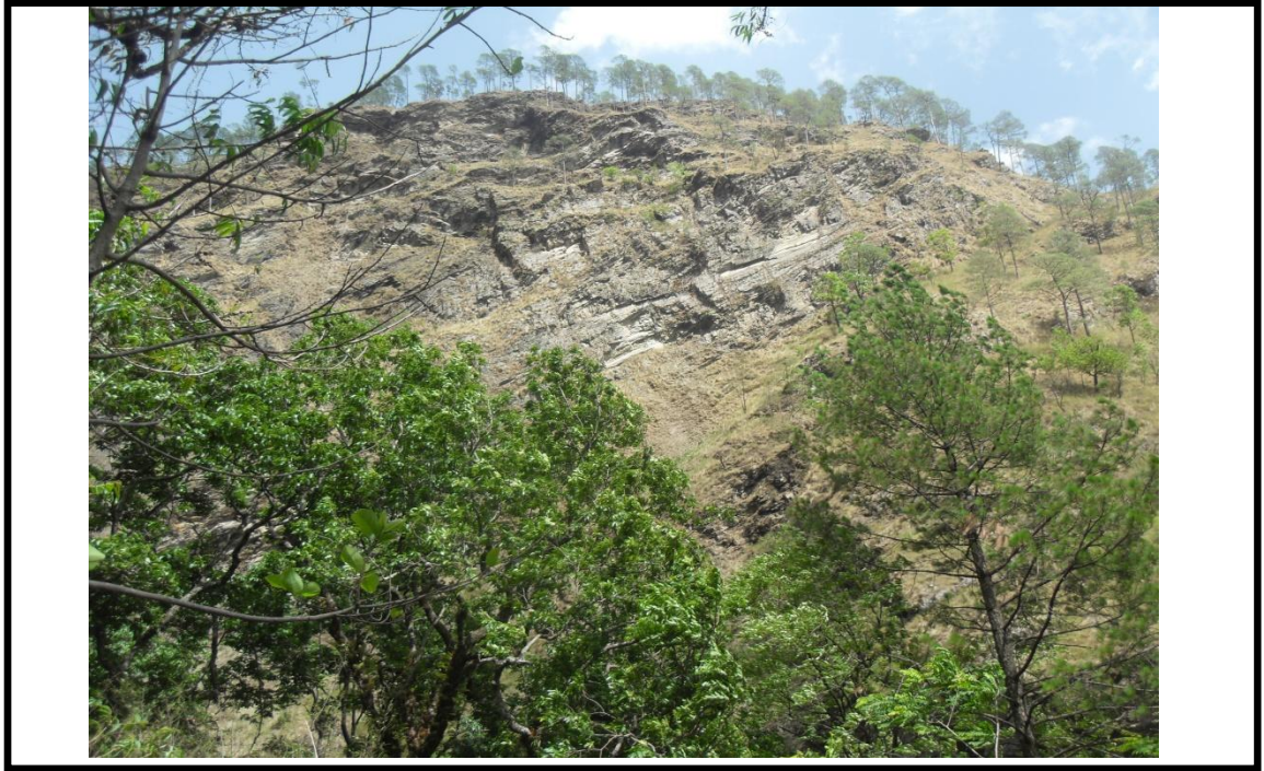
Photograph 7: Bedrocks observed in the Powerhouse Area
