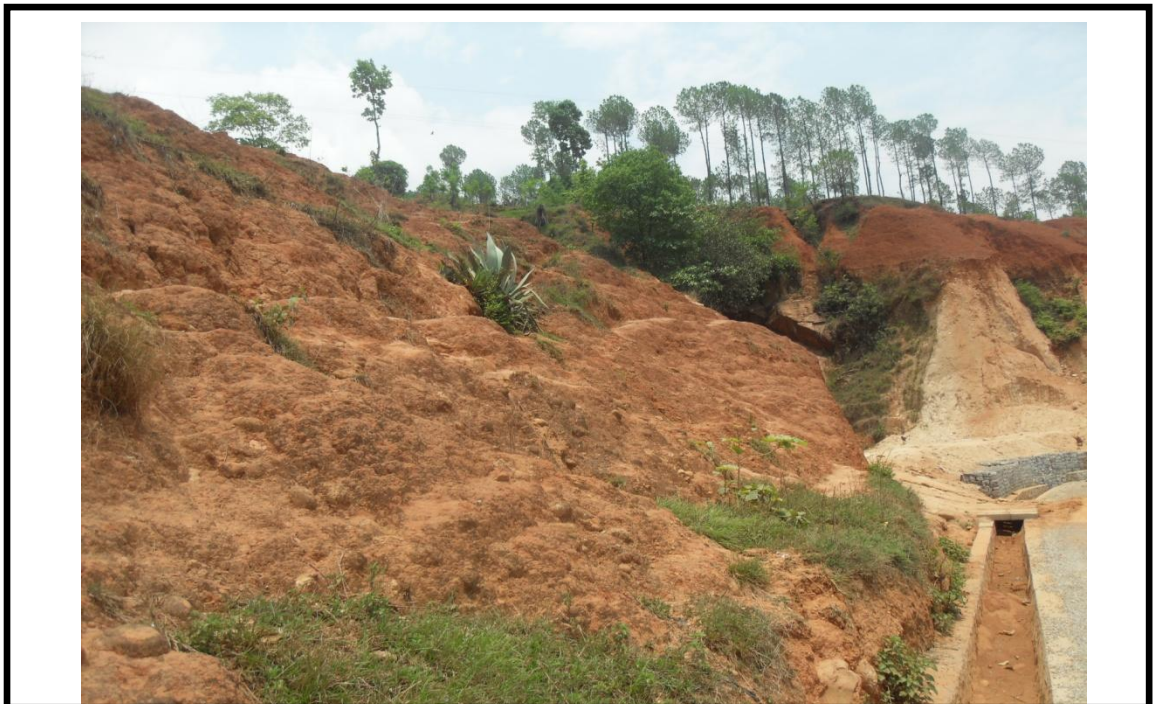
Photograph 10: Red clay deposit along the road section at Battar village
