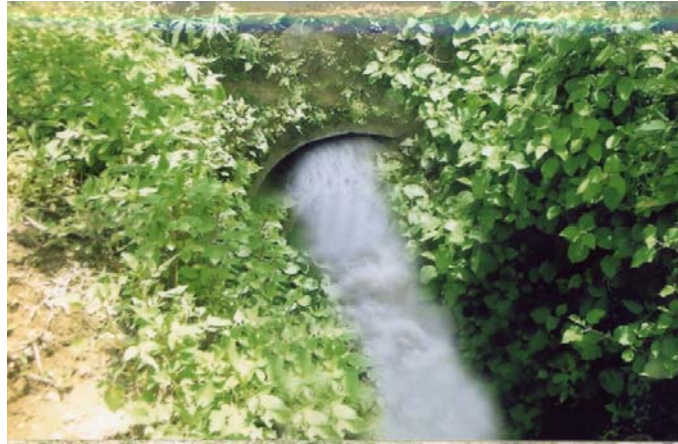
Overflow of drains into the lake.
