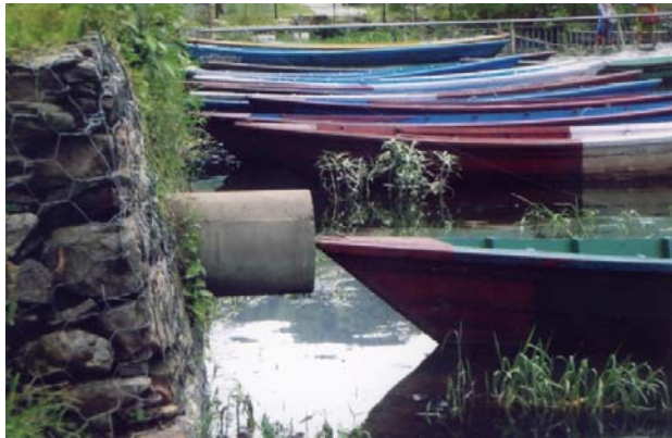
Sewage system connects into the lake.
