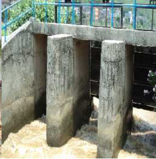
Irrigation canal in Butwal
