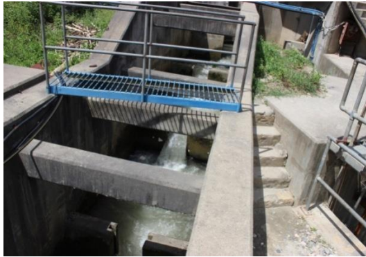
Fig: 1 Fish ladder in dam
