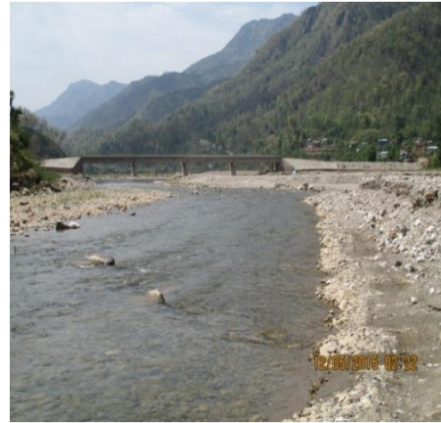
Bridge of Sharada River
