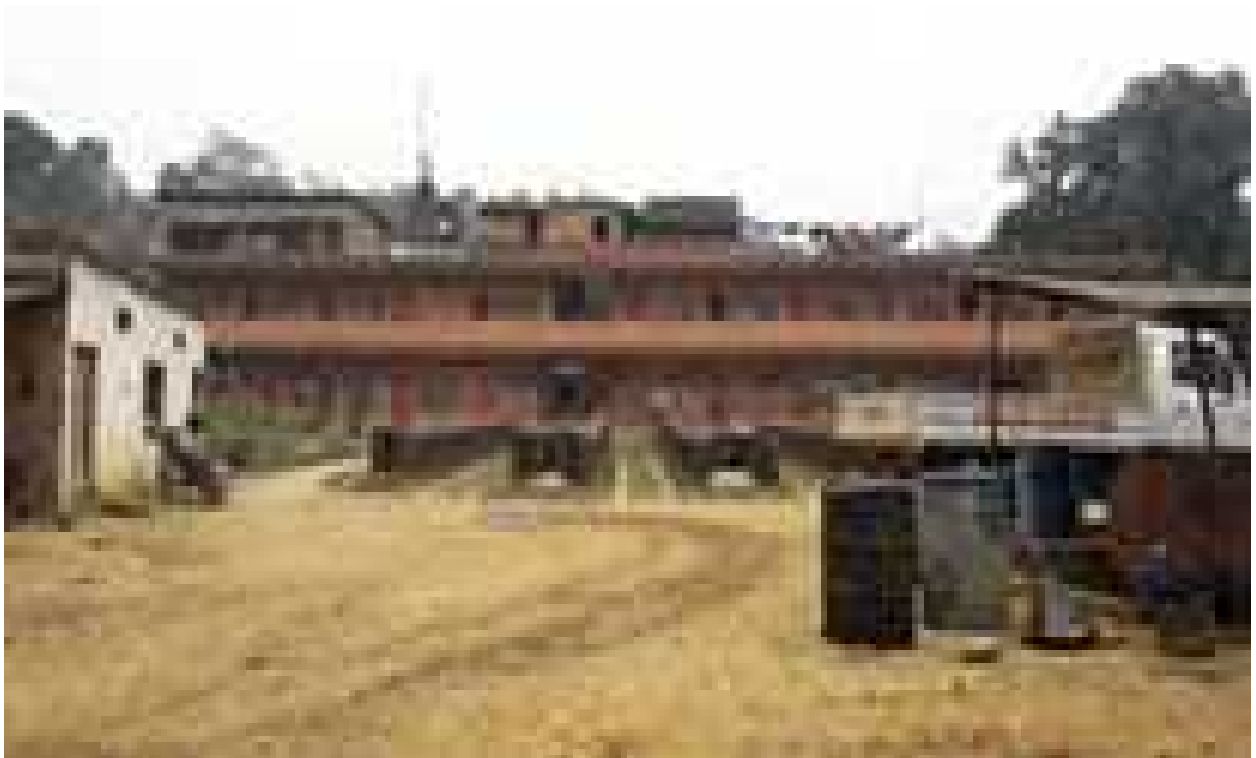
Quarter for labourers in the Brick factory
