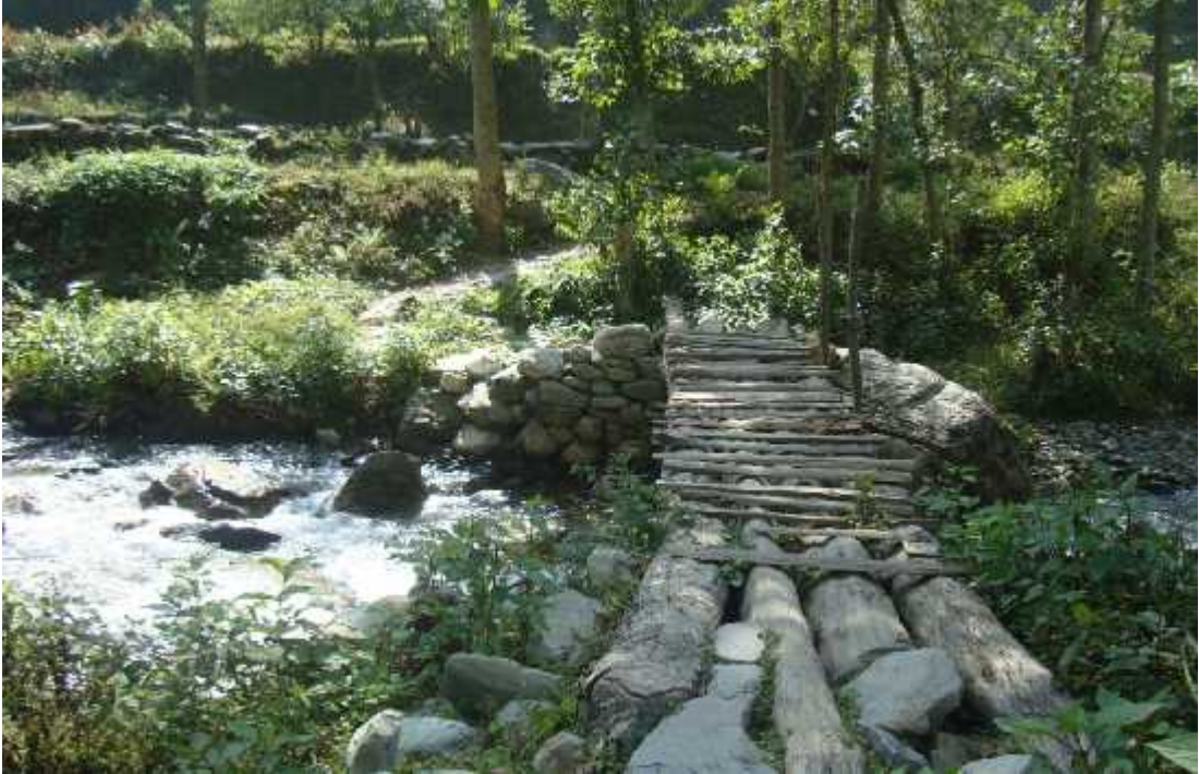
Local Bridge of Gotikhel
