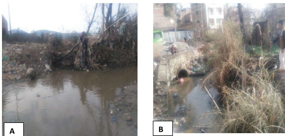
Figure 14: Unplanned Drainage (A) around 100M West of Siddhi Memorial Hospital and Mismanagement of River (B) at Chyamasing East of Bridge
