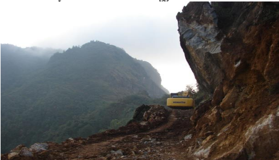
K: Road Construction near cliff.
