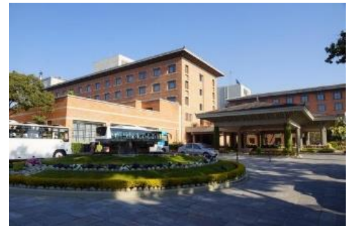
Figure 60: The building after the facade relifting in 1990s
