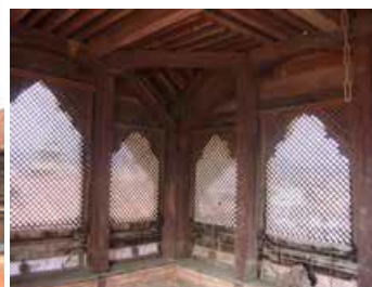
Figure 37: Decorative struts with snake motif supporting curve roof, 2019 and Wooden frame structure supporting the roof, 2017
