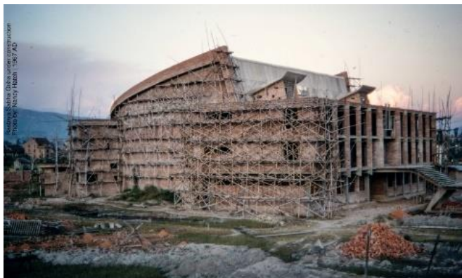
Figure 65: Construction of Rastriya Sabha Griha, 1967
