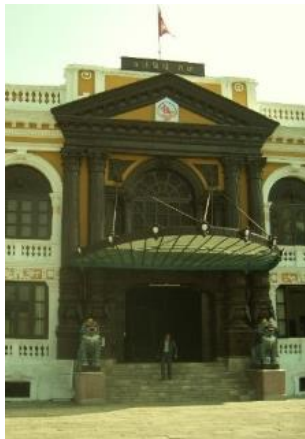
Figure 56: Metal canopy on front façade
