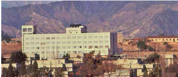
Figure 61: The regular modern facade of the hotel Soaltee, circa 1966
