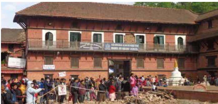
Figure 29: Front facade of Bahadur Shah Hall building (The long projecting wooden balcony along the hall and two-storey high gate at the center to allow elephants to enter)
