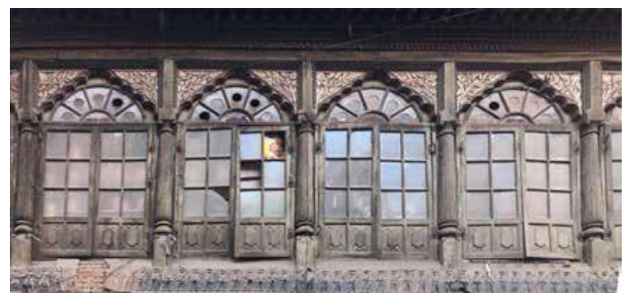
Figure 38: The elaborate decoration on the window posts and bracket and unique army parade
