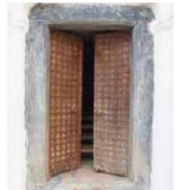
Figure 41: The wooden door panels are provided with metal straps and nails, 2017
