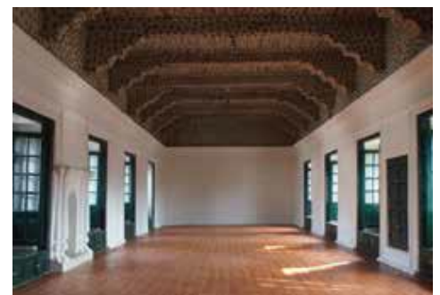
Figure 39: The Bahadur Shah hall (wooden beams, supported by the projecting brackets)
