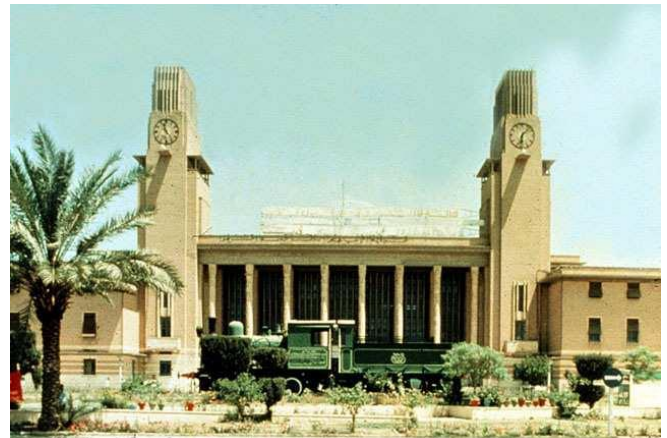
Figure 15: Baghdad's Rail Station
