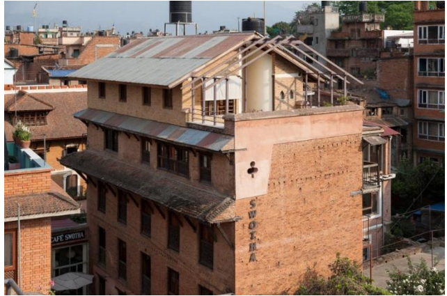
Figure 46: External view of swotha traditional house
