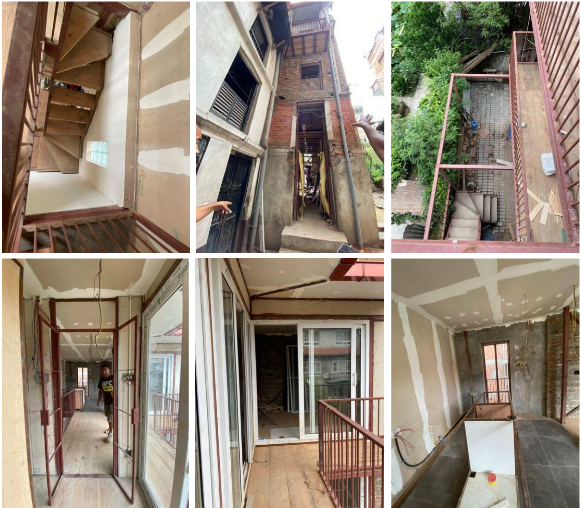
Figure 39: Under construction guest house project of cosy nepal
