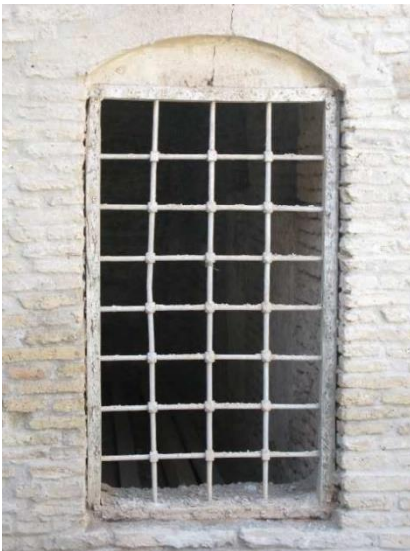
Figure13:A Typical window
