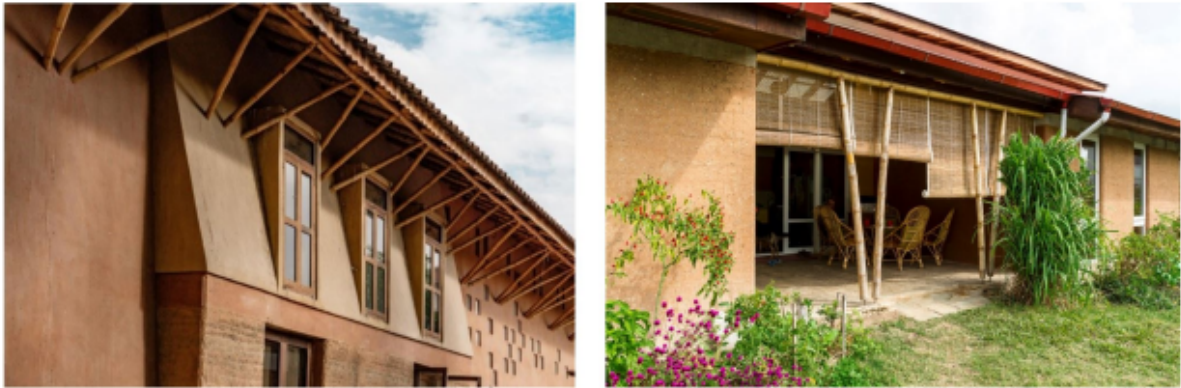
Figure 1: Two Rammed earth structures:(Madan Pustakalaya and Matoghar)
