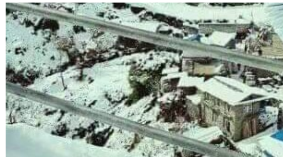
Figure 3.12 Flat and Sloped roof in snow
