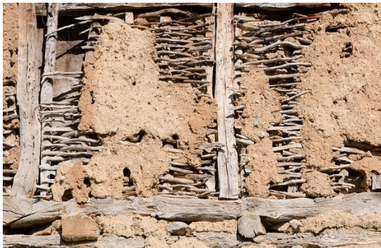
Figure 2.5 Details of wattle and daub
