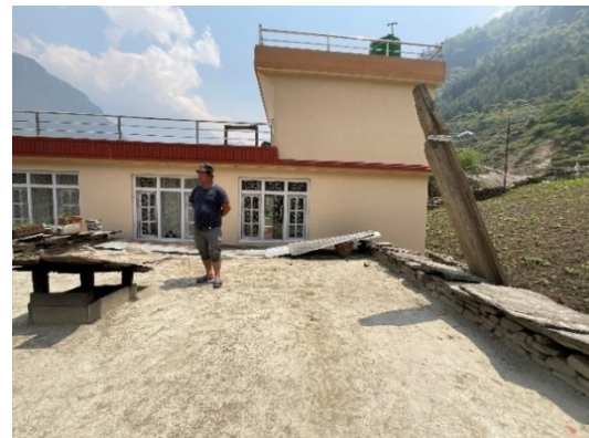
Figure 3.26 House D - Roof
