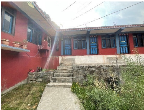
Figure 3.31 House F- Outside
