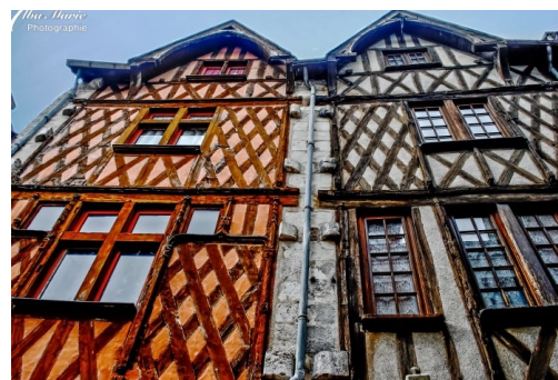
Figure 1.4 Wattle and Daub, France Source: (WordPress, 2016)
