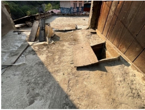
Figure 3.23 House C- roof
