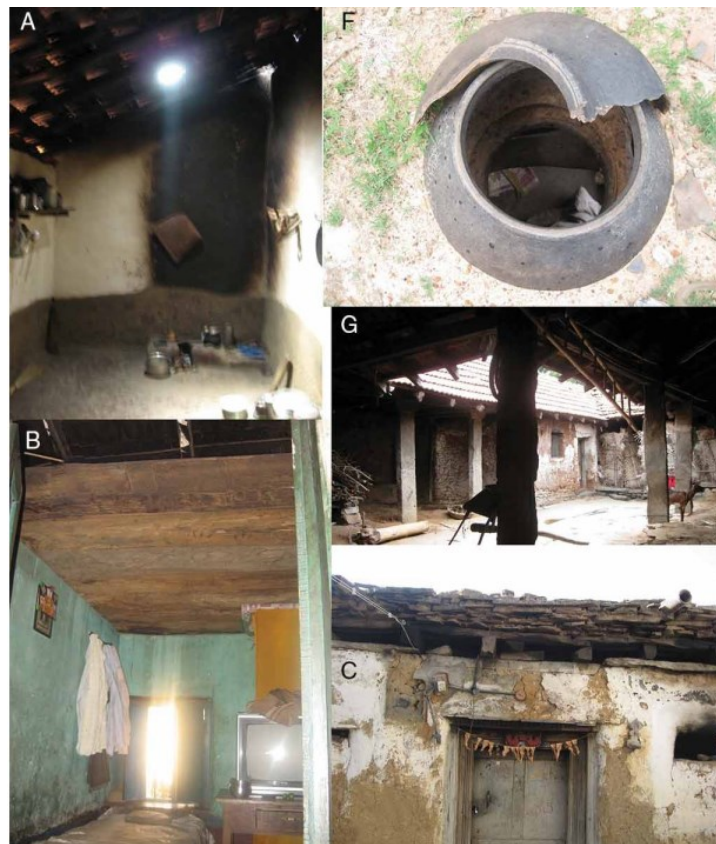
Figure 2.37 Materials used inside and outside the building
