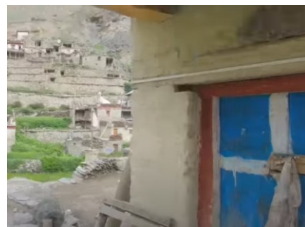
Figure 3.7Mud used as outer protection
