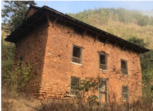
Figure 2.9 2-story SMM shelter Source : (HRRP, 2018)
