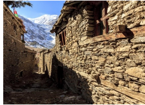
Figure 2.12 Manang (mud as binding material)
