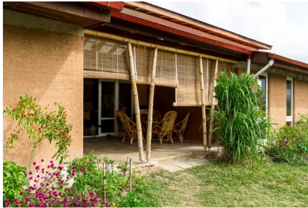
Figure 2.8 Modern Rammed earth structure -Matoghar
