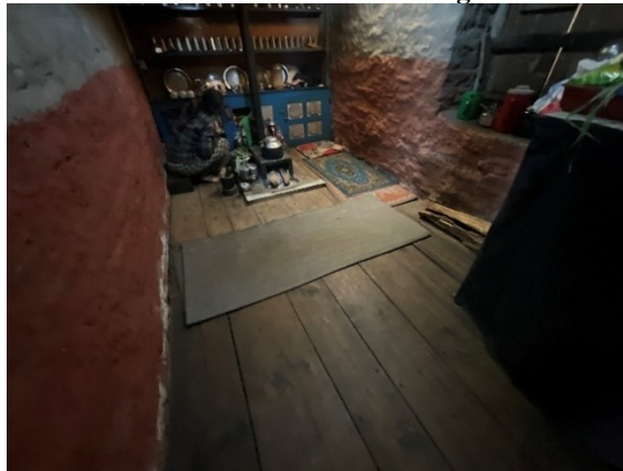
Figure 3.37 Kitchen area SMM with mud plaster
