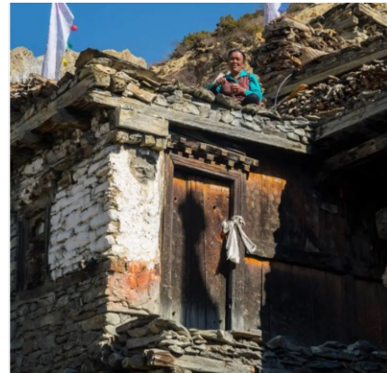
Figure 3.5 Mud Used as Mortar
