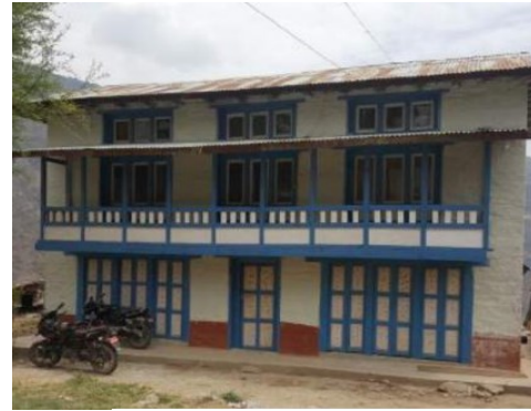
Figure 2.10 SMM with mud plaster – Solukhumbu Source : (EFIT,2019)
