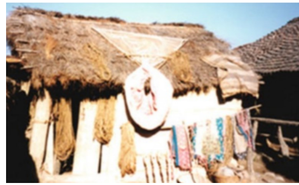
Figure 2.16 Banke Thatched Roof Mud House
