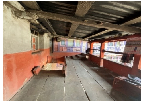
Figure 3.24 House D - Verandah
