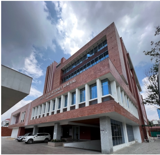
Figure 49: South west view
