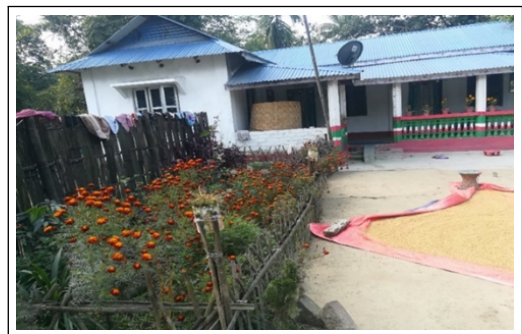
Figure 8: Santhal RCC house with CGI sheet
