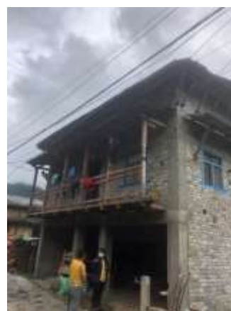
Figure 18 Hybrid structure in Thabang
