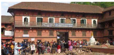
Figure 4.7: Front facade of Bahadur Shah Hall building (The long projecting wooden balcony along the hall and two-storey high gate at the center to allow elephants to enter)
