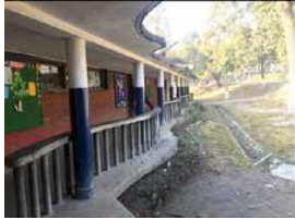
Figure 4.34: The playful walkway along with flowing concrete slab edge Source: (Nepal, 2020)
