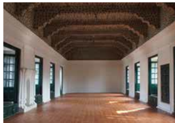
Figure 4.8: The Bahadur Shah hall (wooden beams, supported by the projecting brackets)
