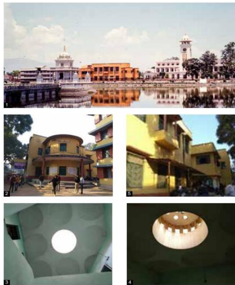
Figure 4.28: view of Saraswati sadan behind Ranipokhari , projecting concrete slab, use of skylight and the ceiling design in the lower lobby of the northern wing with cantilever balconies and projections
