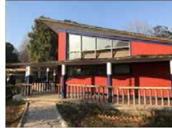
Figure 4.32: The clerestory windows below the winged concrete slab Source: (Nepal, 2020)
