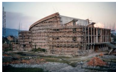
Figure 4.40: Construction of Rastriya Sabha Griha, 1967 Source: (Nepal, 2020)
