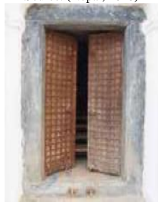
Figure 4.14: The wooden door panels are provided with metal straps and nails, 2017
