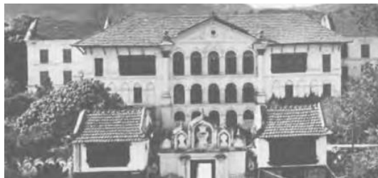
Figure 4.10: Front facade of Chhauni Durbar with arched french windows and corithian column, 1975
