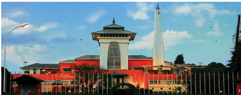
Figure 4.44: Front facade with the two towers dominating the façade
