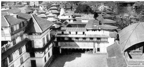
Figure 4.15: Aerial view of Sisha Baithak ,1920s Source: (Nepal, 2020)
