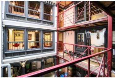
Figure 5.15: Blend of traditional and modern construction
