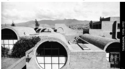
Figure 5.23: Cylindrical brick vault structure, Taragaon Source: (2) Valerie Messina "Über Carl Pruscha" - YouTube
