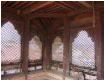
Figure 4.4: Wooden frame structure supporting the roof, 2017 Source: (Nepal, 2020)
