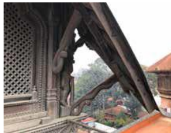
Figure 4.3: Decorative struts with snake motif supporting curve roof, 2019 Source: (Nepal, 2020)
