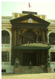
Figure 4.26: Metal canopy on front façade
