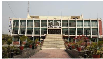
Figure 4.39: Rastriya Sabha Griha Source: https://spacesnepalblog.wordpress.com/2018/06/12/nepals-first-architect/
