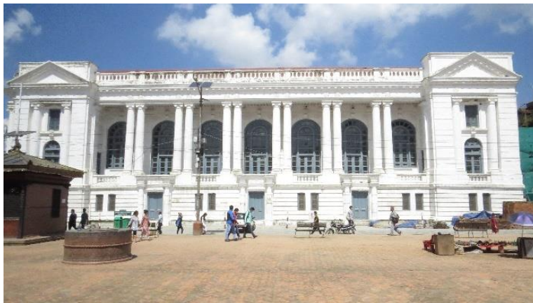
Figure 4.23: South Facade of Gaddhi Baithak Source: https://www.flickr.com/
