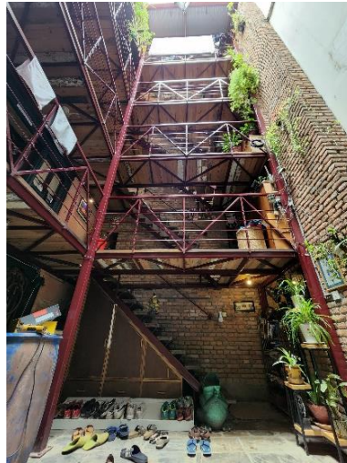
Figure 5.17: Metal structure for staircase block Source: field visit
