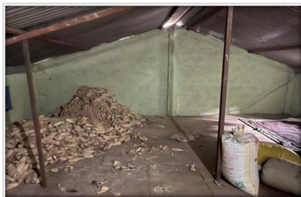
Figure 36 Attic for Storage in Namuna Basti
