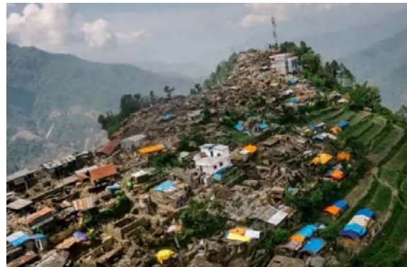
Figure 8 Barpark after 2015 Earthquake (Source: ekantipur.com)
