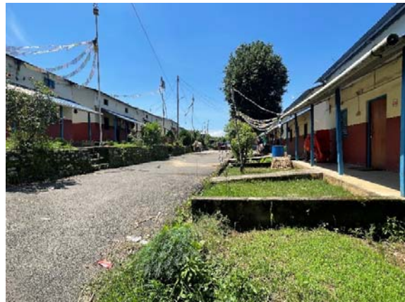
Figure 57 Bituminous Road in Namuna Basti
