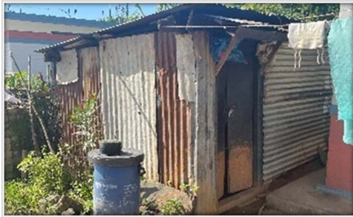
Figure 51 Temporary Shelter for Storage
