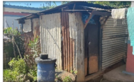
Figure 11: Temporary Shelter for Storage
