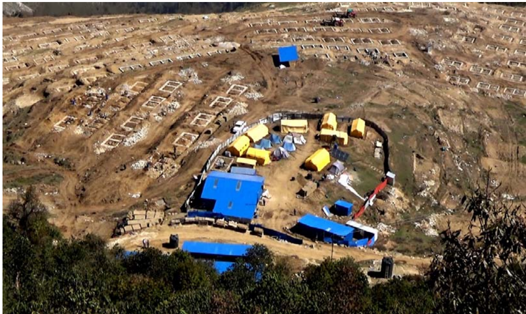
Figure 13 Settlement under construction of Ghupsipakha (nrna.org)
