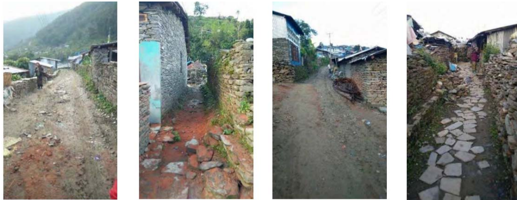
Figure 9 Walkways of Laprak After earthquake (Source: Resettlement planning project, 2017)
