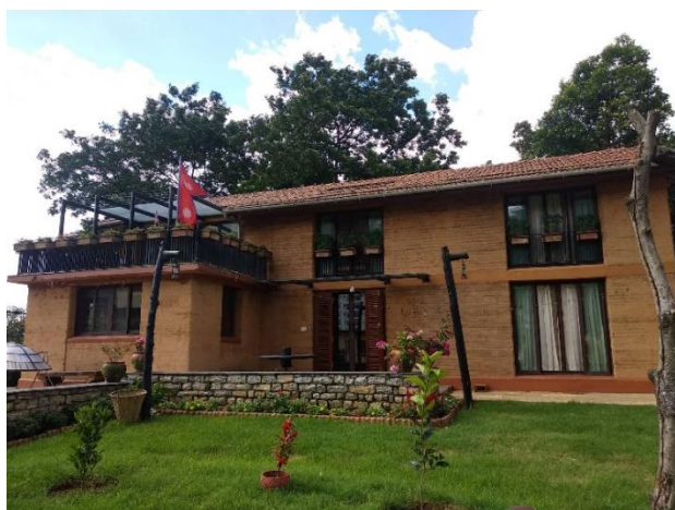
Figure 117: Use of rammed earth, cement plater
