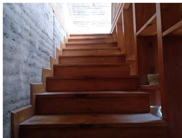
Figure 118: Use of timber, mud plaster
