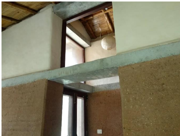
Figure 77: Use of earth, cement plaster
