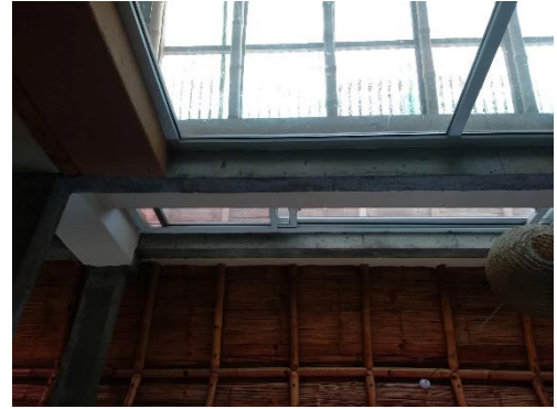
Figure 72: Mato ghar Ceiling opening
