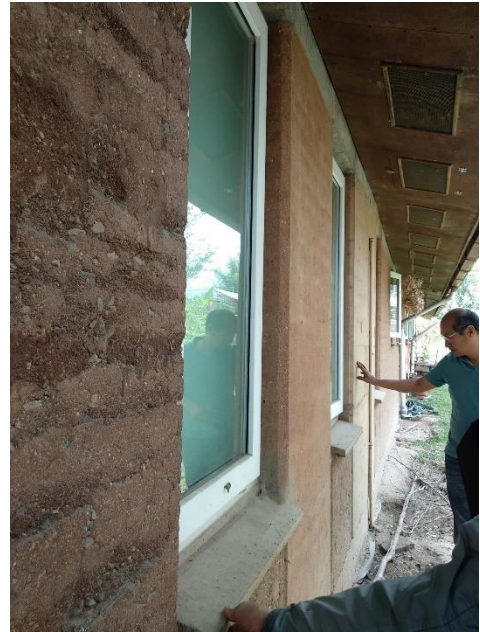
Figure 51: Use of rammed earth techniques
