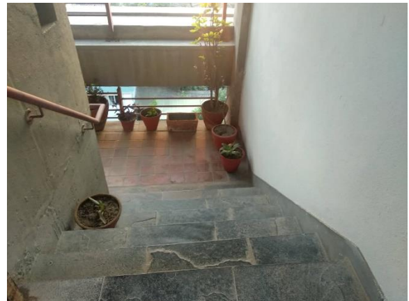
Figure 89: Exposed concrete, wall without plaster
