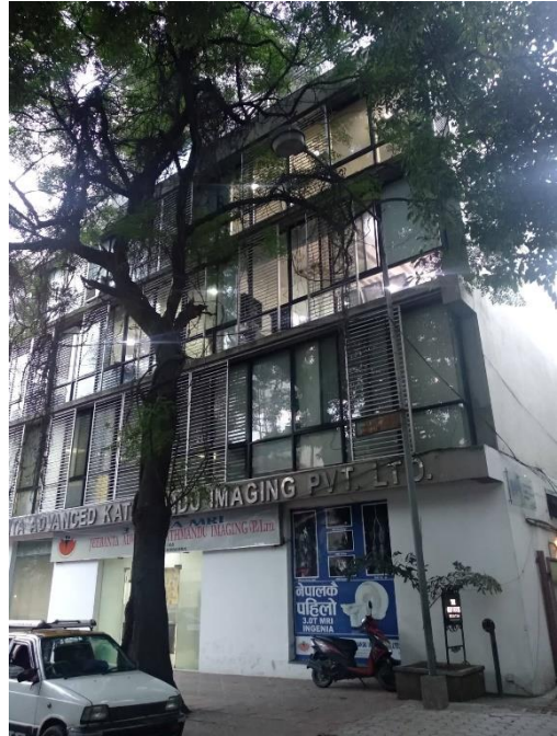
Figure 80: Sura building of Durbarmarg
