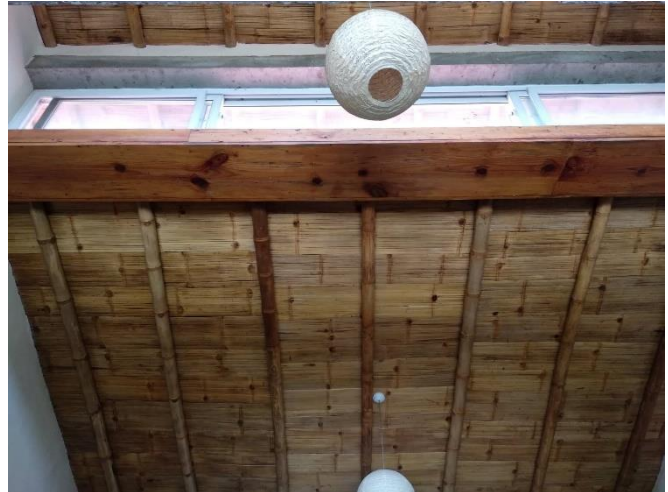
Figure 54: Straw roof with bamboo rafter
