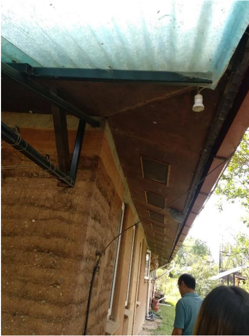
Figure 53: Natural ventilation through roof
