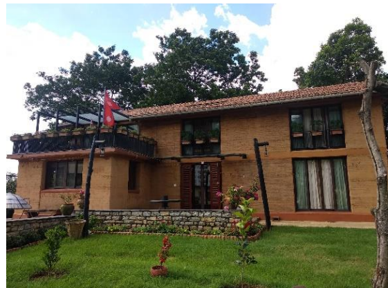
Figure 106: Gutter for rainwater harvesting
