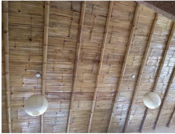
Figure 70: Passive cooling technique for roof
