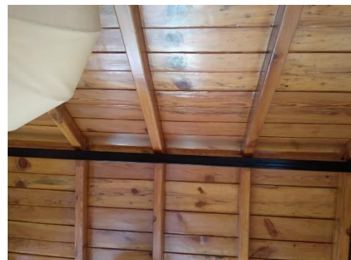
Figure 108: Roof wooden planks
