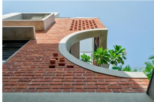
Figure 22: Opening on south west corner
