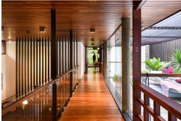
Figure 34: Wooden ceiling for thermal insulation
