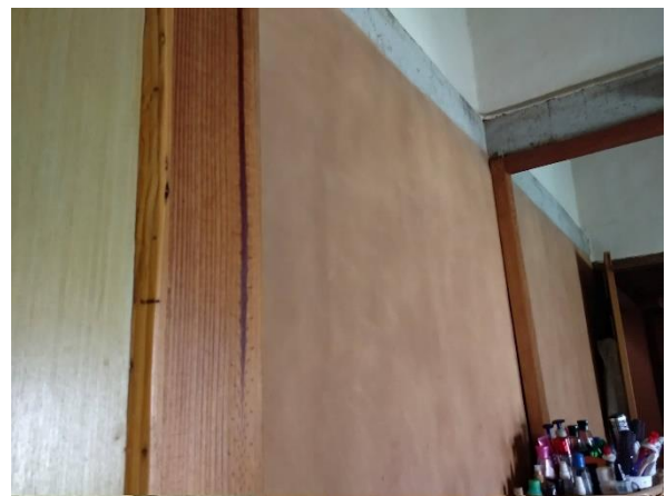
Figure 76: Use of timber, mud plaster
