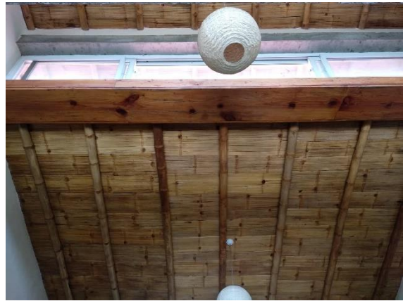
Figure 56: Skylight of top floor
