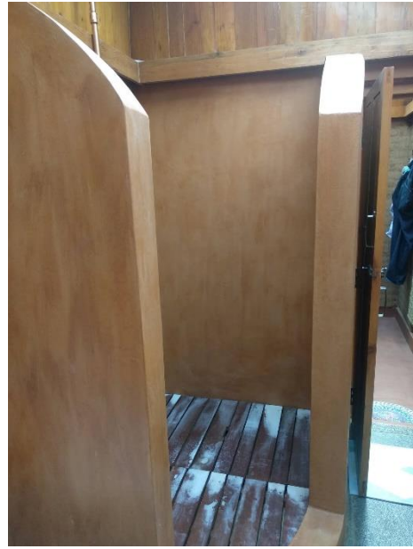
Figure 109: Flooring in bathroom
