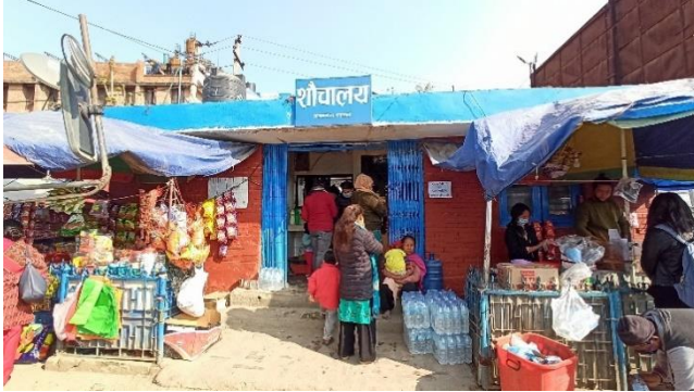
Figure 3-18 Inaccessible Public Toilet
