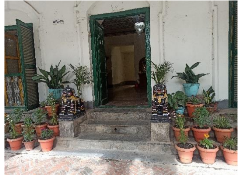
Figure 3-45 Inaccessible Entrance at Admin Block
