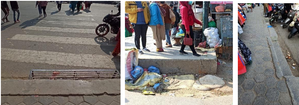
Figure 3-13 No guides on the crosswalk
