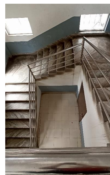
Figure 3-50 Inaccessible Upper Floors
