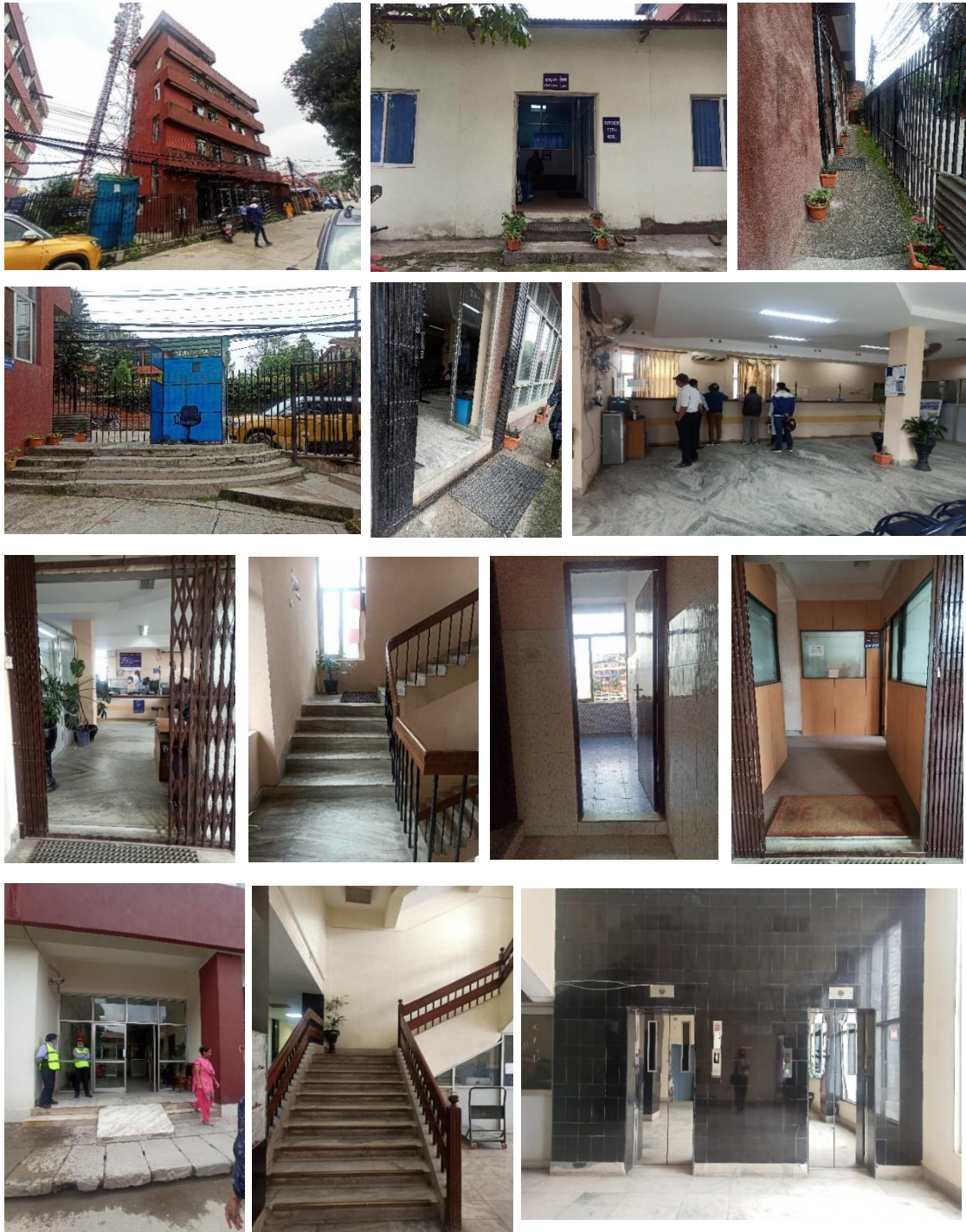
Figure 3-48 Nepal Telecom Office, Jawalakhel
