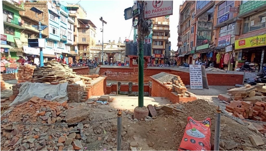
Figure 3-9 Inaccessible drinking water facility
