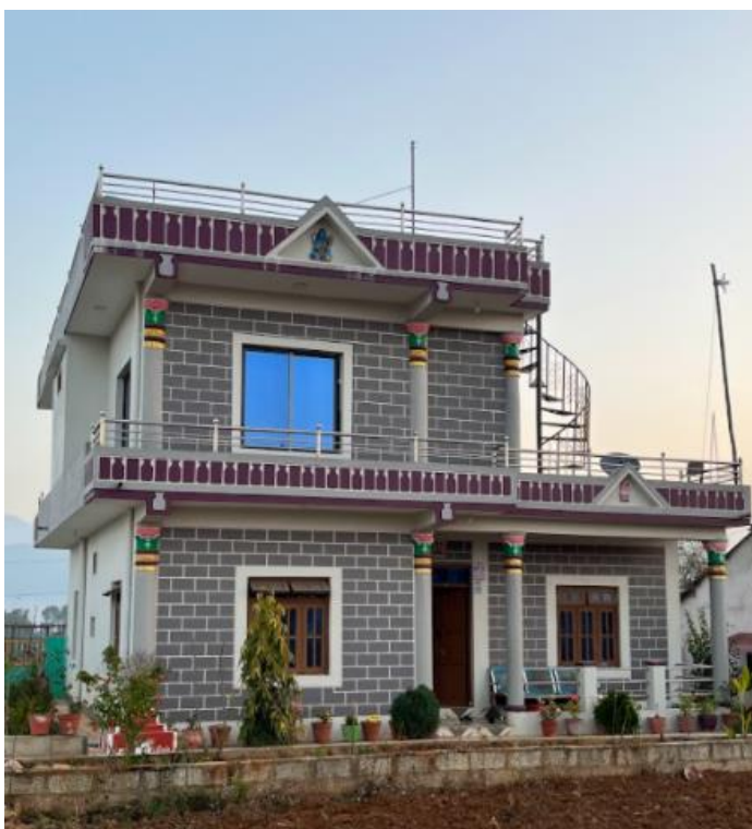
Figure 6-1 building selected for applying design strategies which has been recommended
