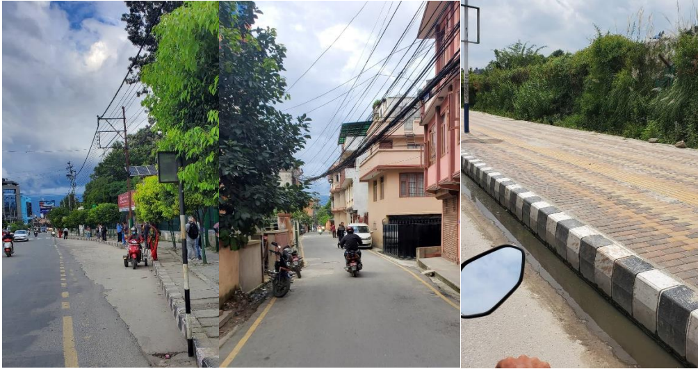
Photo B.6 Typical Road Infrastructure in Kathmandu
