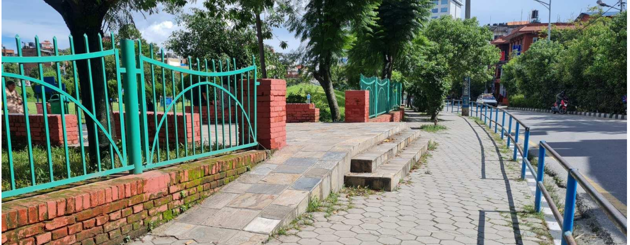
Figure 8: Entry way to Narayanchaur
