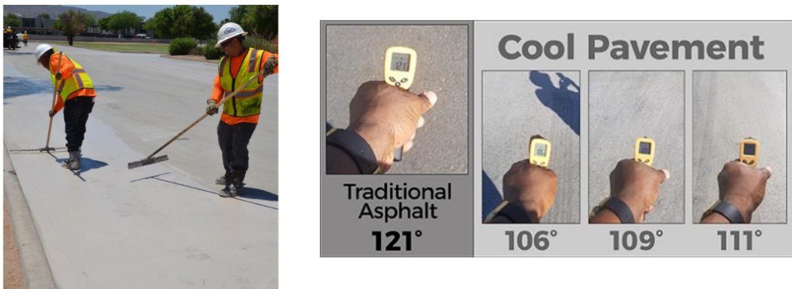
Figure 15: Phoenix city workers are covering streets with a cool surface as part of a pilot project that Arizona State University is evaluating
