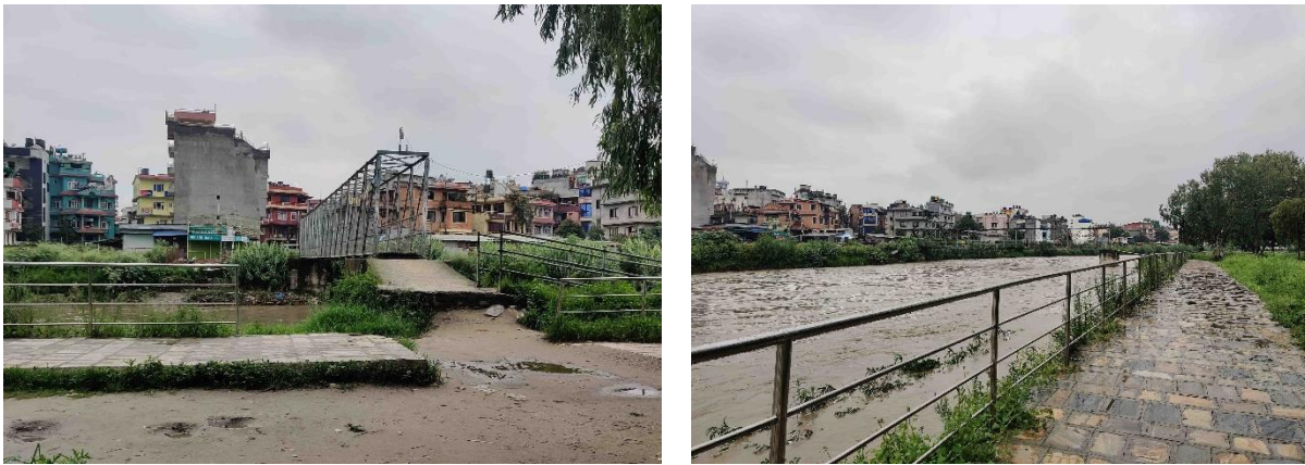
Figure 10: Commuter bridge and walkway adjacent to the river
