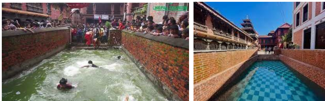
Figure 27: new pond construction at temple space
