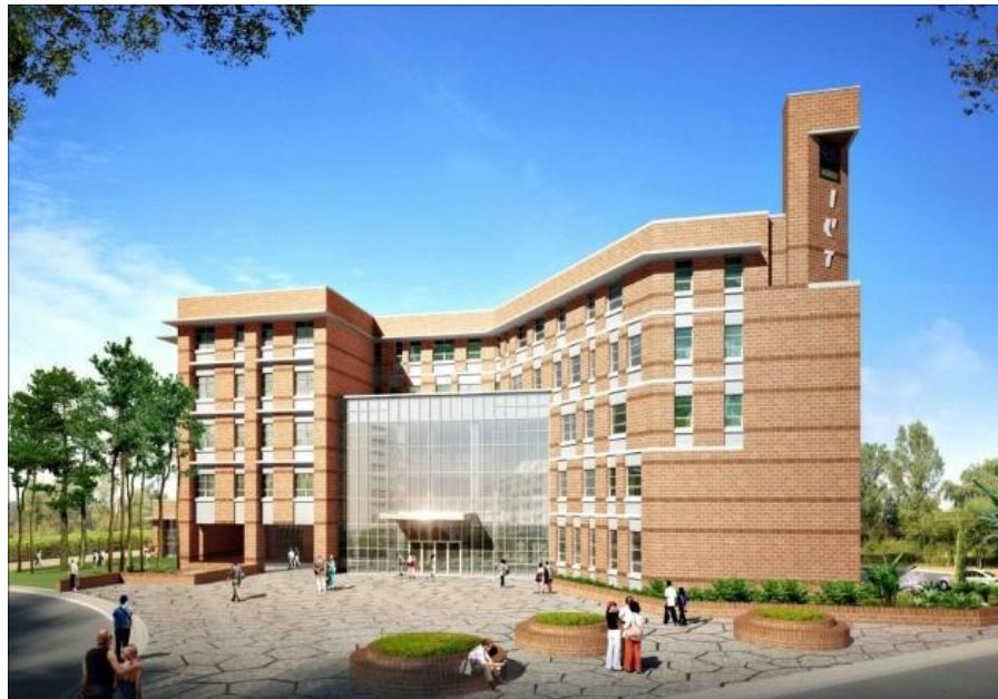
Figure1: ICTC Building, Pulchowk Engineering College
