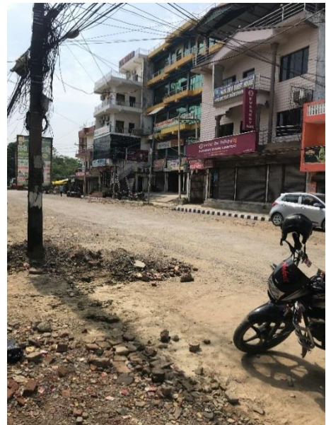
Figure 4. 4 street view towards north
