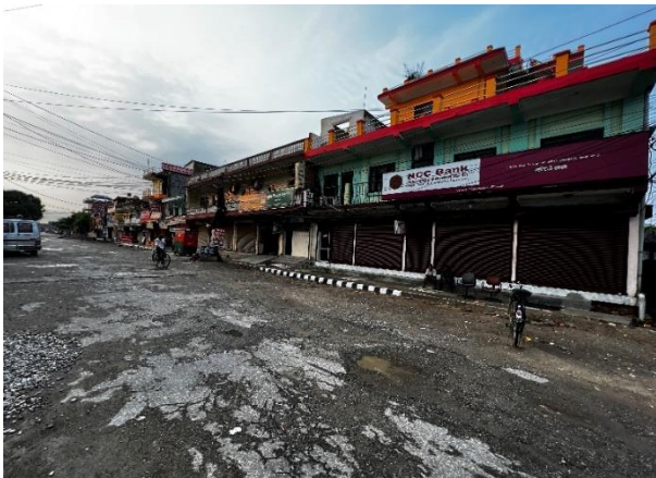
Figure 4. 5 street view towards south
