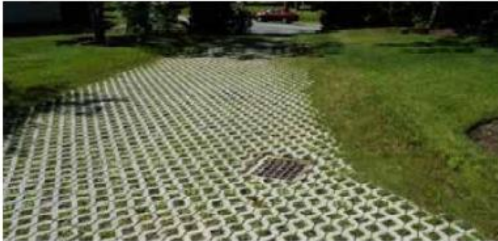
Figure 2-37 Honeycomb Pavers allow water permeation Source: 2017 State of New Jersey Complete Streets Design Guide
