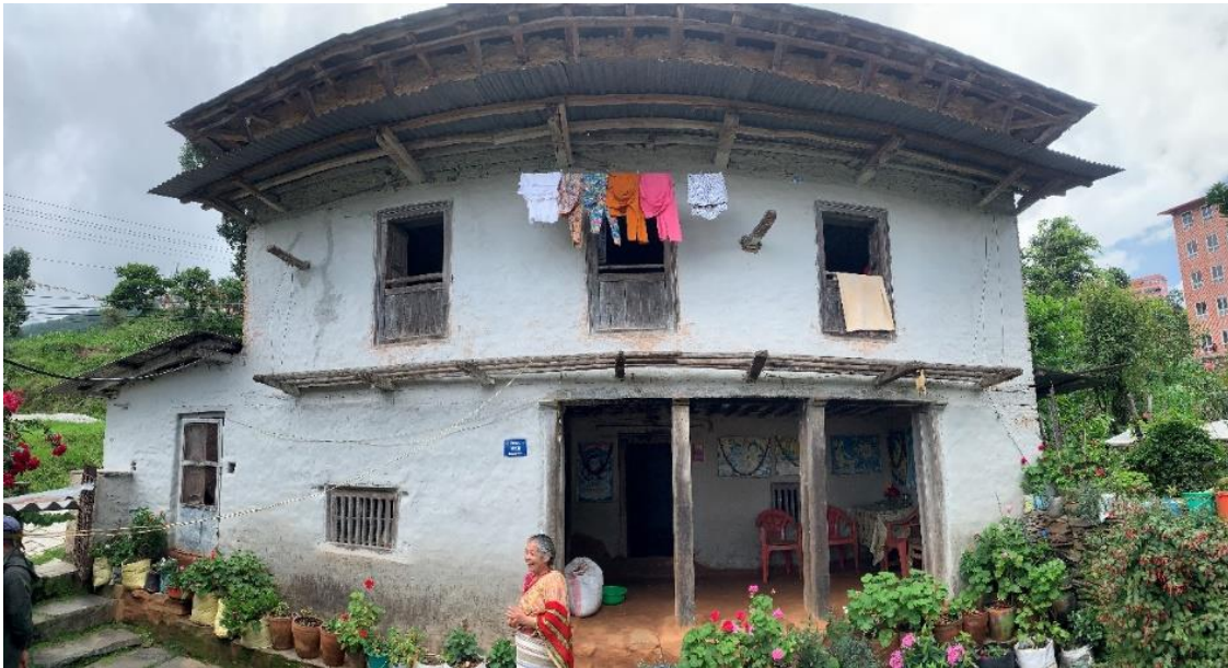
Figure 44 Case 1: Traditional House of Dolakha town
