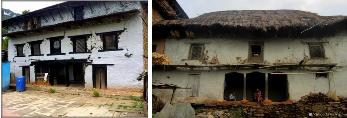
Figure 38 South Facing House (Source: Anil Chandra Shrestha)
