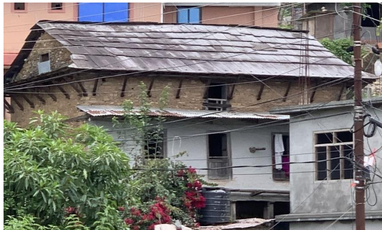
Figure 60 Rough textured Slate roof
