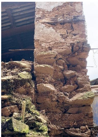
Figure 53 Stone Wall with mud mortar
