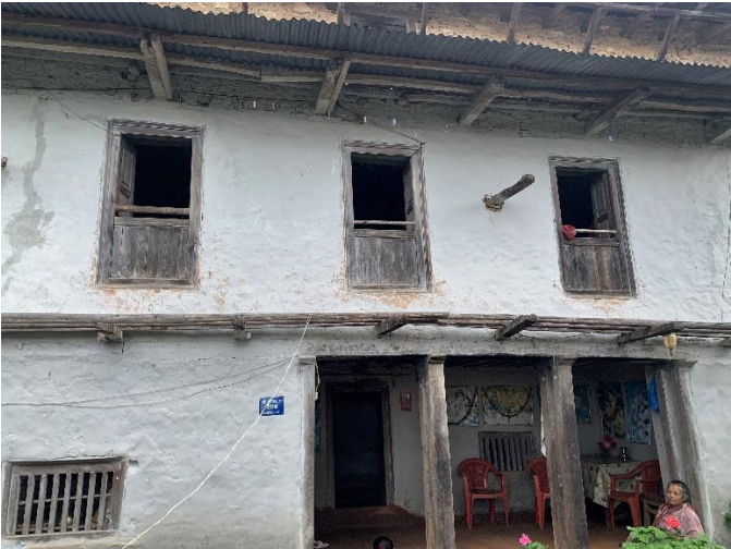
Figure 51 Fenestration on south wall
