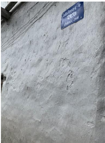
Figure 59 Irregular and rough wall surface
