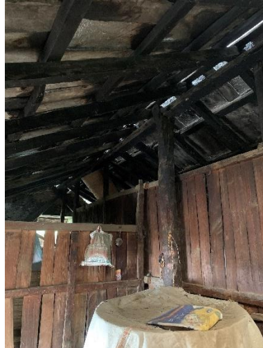
Figure 57 Slate roof Supported by timber structure
