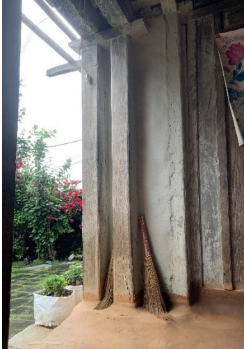
Figure 56 Timber as Structural member
