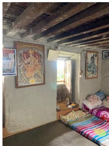
Figure 54 Internal wall surface rendered with Kamero mato
