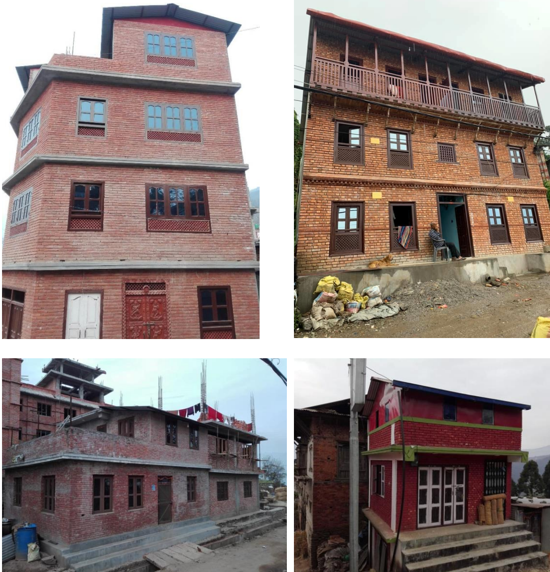
Figure 41 Residential Buildings after Earthquake 2015
