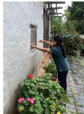
Figure 55 External wall surface rendered with Kamero mato
