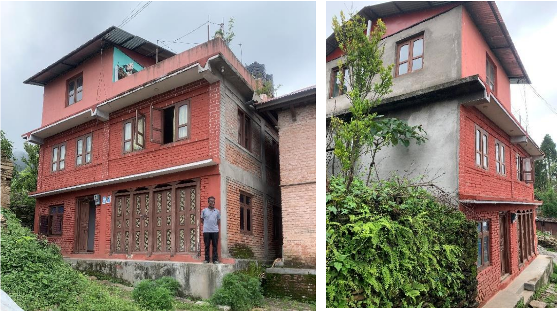
Figure 63 Case 2: Post Disaster Reconstructed Building
