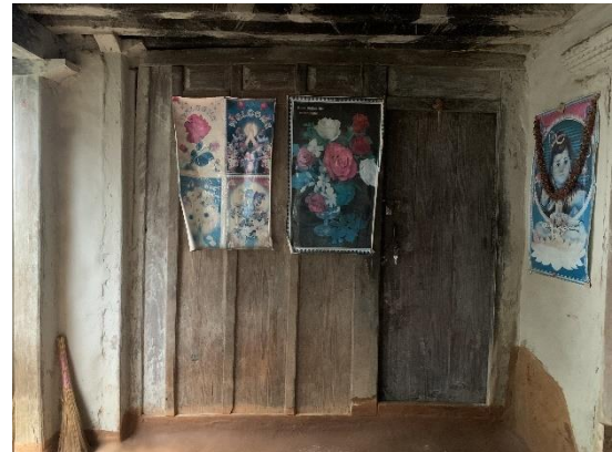
Figure 49 Timber boards for Partition wall
