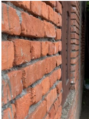
Figure 67 External brick facade
