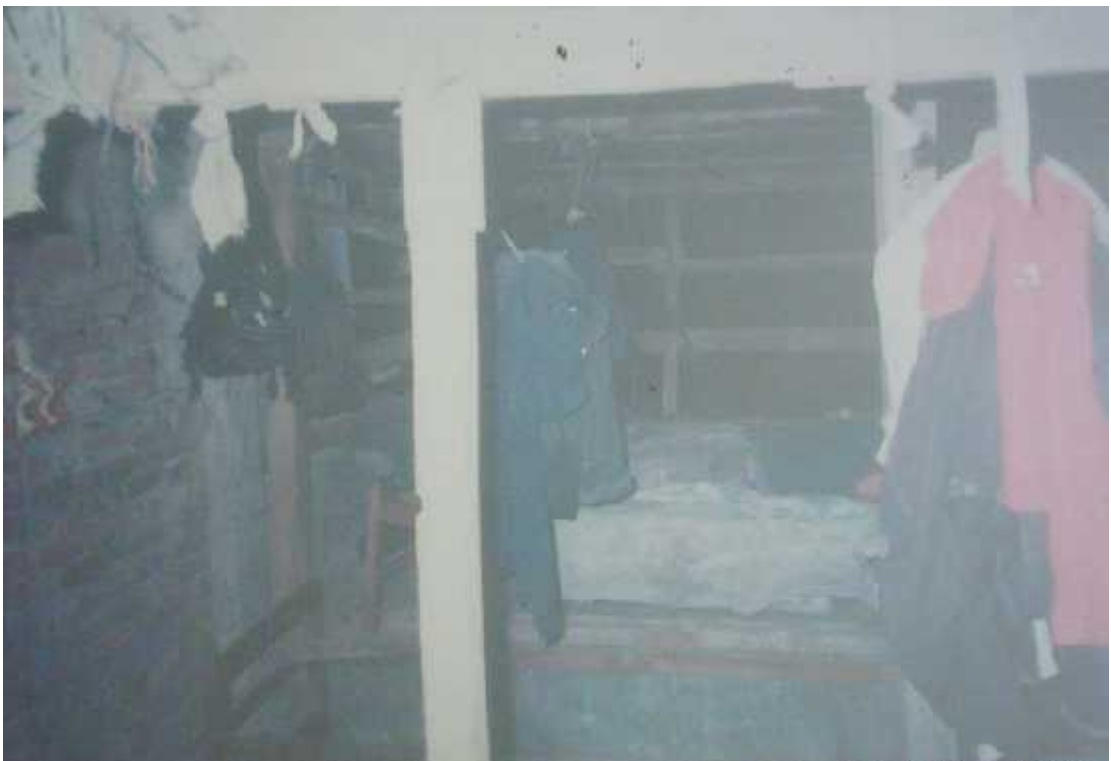
Condition of bed for child labour in the hotel. It is at the top of the hotel under the open sky.
