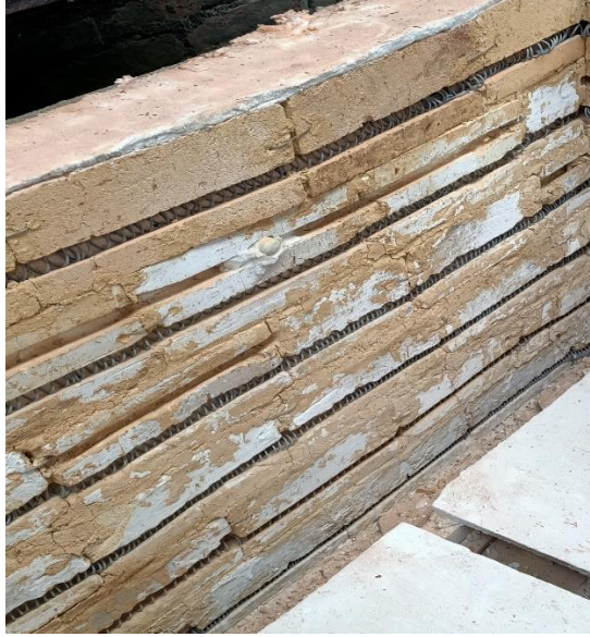
Figure 3.3: Furnace wall with the Kanthal wire and thermocouple
