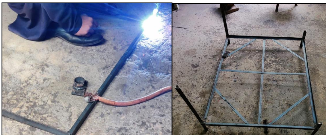
Figure 3.10: SS support structure fabrication
