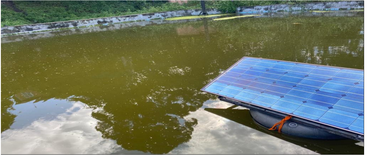
Figure A.3 FSPV System on the site
