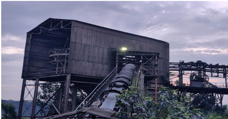
Figure 6-5: Ropeway starting point and hopper
