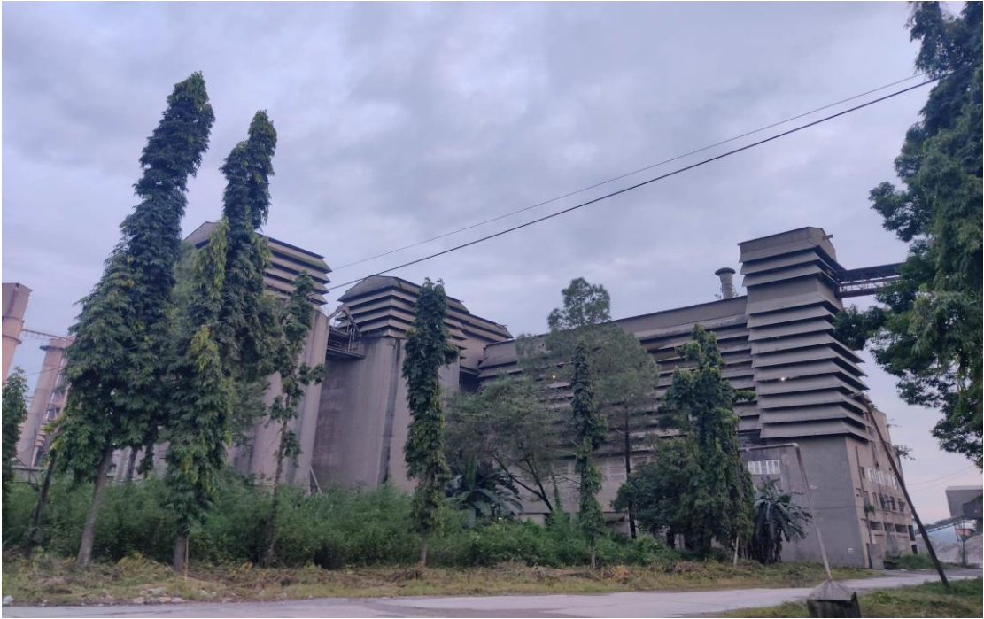
Figure 6-1: Cement mill building
