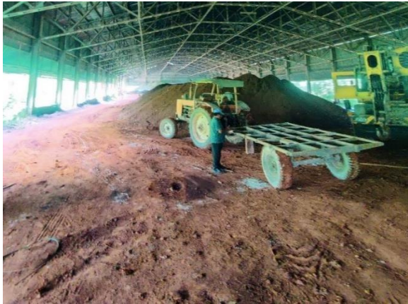
Figure 6-10: Iron ore yard
