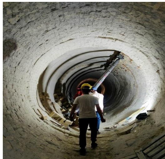
Figure 6-14: Inside of kiln
