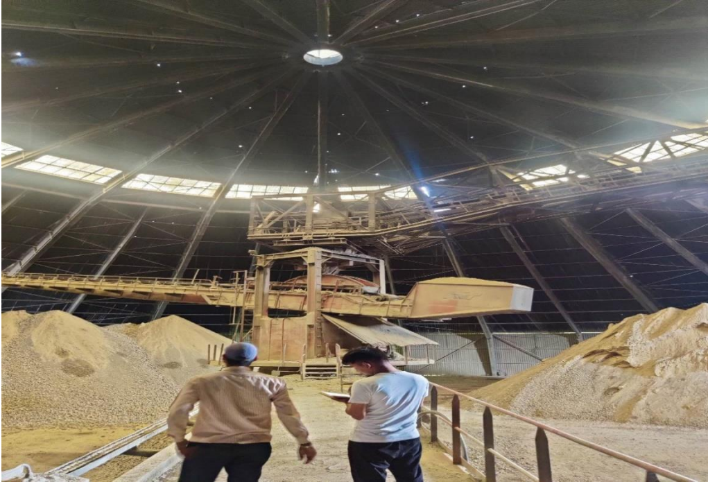
Figure 6-8: Inside of PB hall
