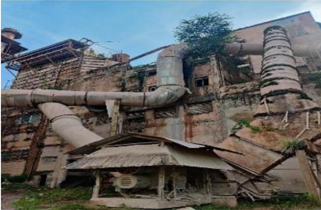
Figure 4-11: Ductway to RABH
