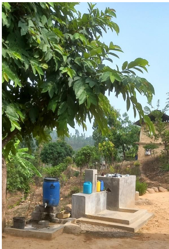
Figure 8: Existing toilet and improved hand washing stations at community
