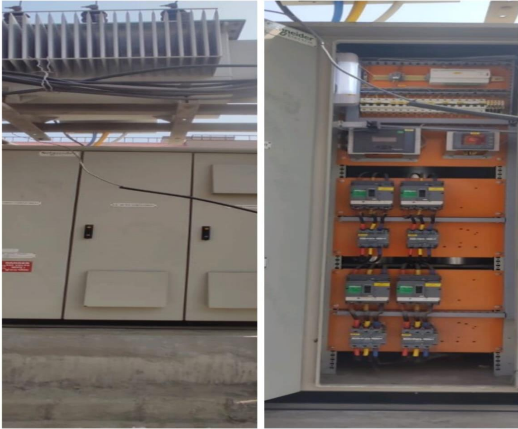
Figure 3.5 Panel for Bess Storage
