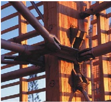
Steel support to the Structure
