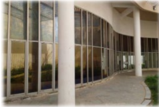
Glazed facade of library
