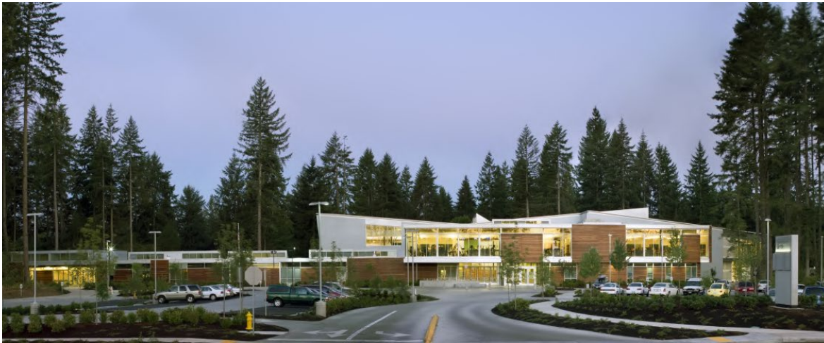
Figure 34 Firstenburg Community Center
